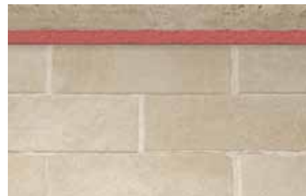
Joint de construction
