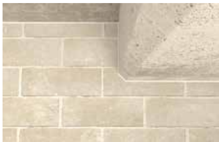
Joint de construction
